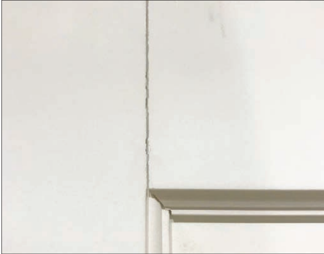
Stile and Rail Separation (Wood Door)
