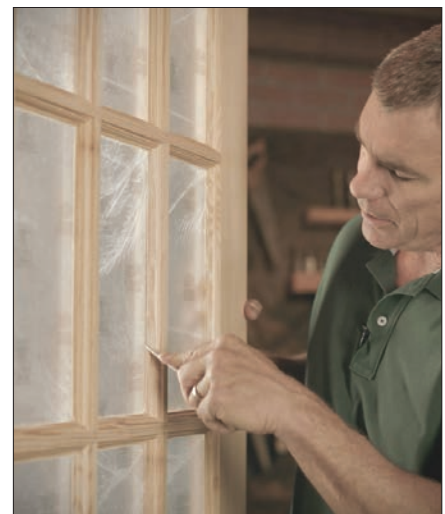
Removing glazing compound
