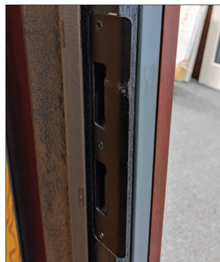
Acceptable hardware wear and tear
