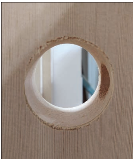
Blowout that can be covered by escutcheon
