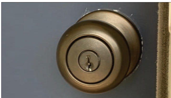
Finish damage caused by use
