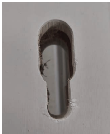
Blowout that can be covered by escutcheon
