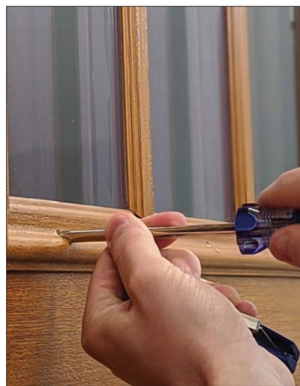
Insert frame screws
