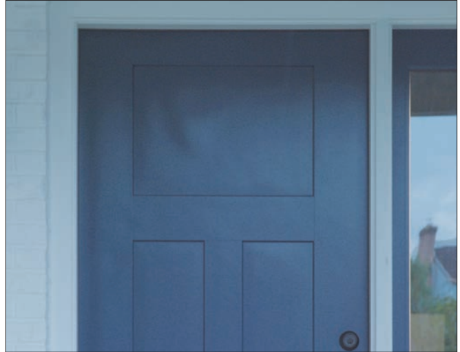
Bubble Defect (Fiberglass Door)
